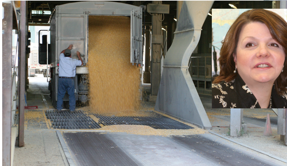
At a corn sweeteners wet grind plant, the bulk weigh scale combines 35-foot and 60-foot scales on either side of a 20-foot pit to accommodate smaller trucks as well as belly-dumpers.
