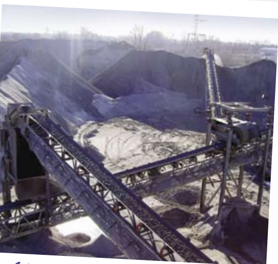
Crisscrossing conveyors of the Beelman Truck Co., Granite City, IL
