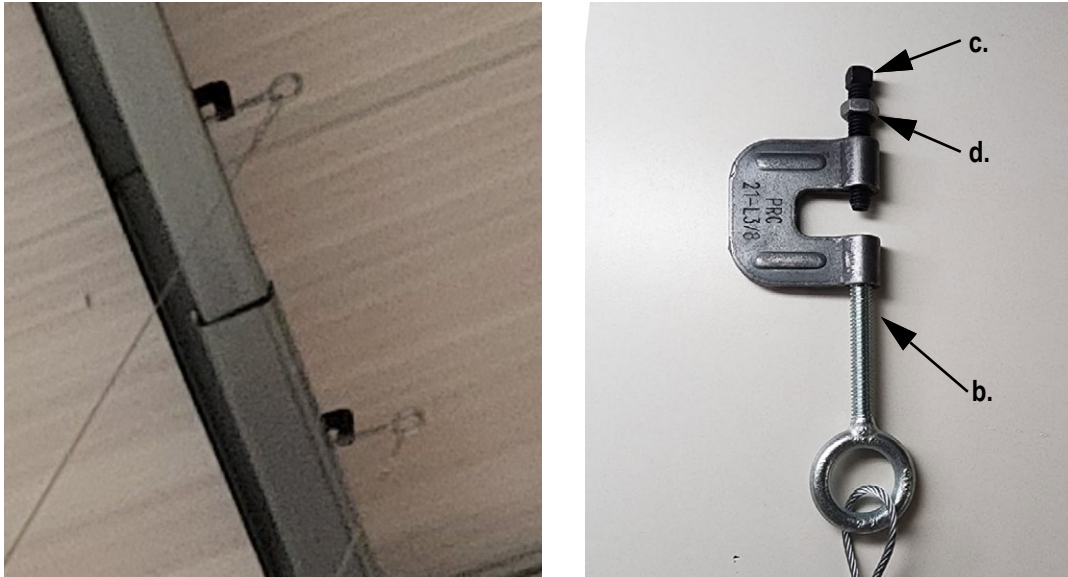
Figure 3. Beam Clamp to Roof Structure
