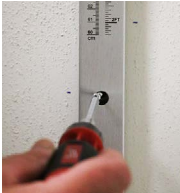
Figure 2-3. Bottom Screw Placement
