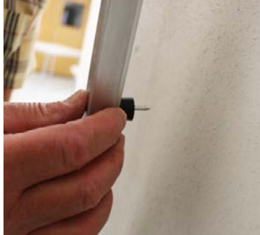
Figure 2-2. Spacer Placement
