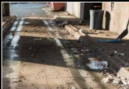
A mix of solid waste chemicals, called "leachate," creates a highly corrosive environment.
