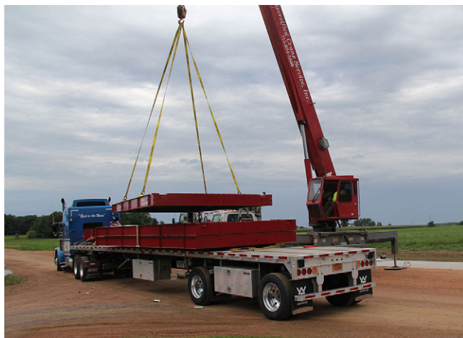
Figure 2-1. Lifting Deck Modules
