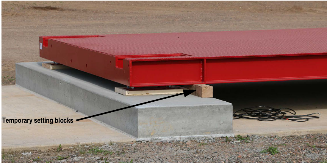
Figure 3-3. Module Positioned on Temporary Setting Blocks
