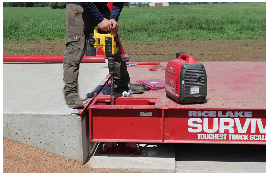
Figure 4-9. Drill Anchor Bolt Holes
