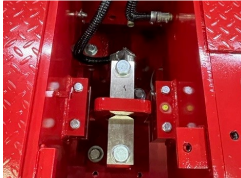
Figure 5-3. Load Cell Pocket Conduit Installed
