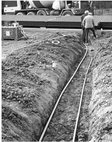
Figure 7-1. Conduit Run in Trench
