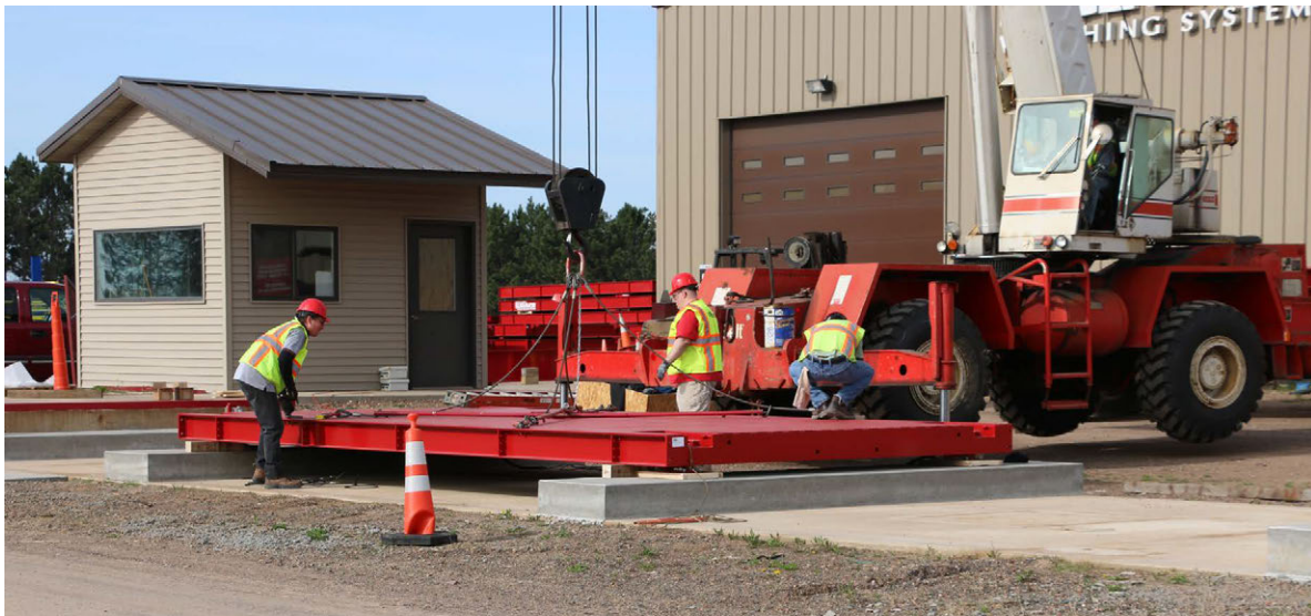
Figure 3-4. Setting Modules in Place
