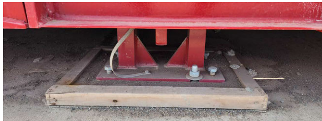
Figure 4-13. Framed and Grouted Baseplate
