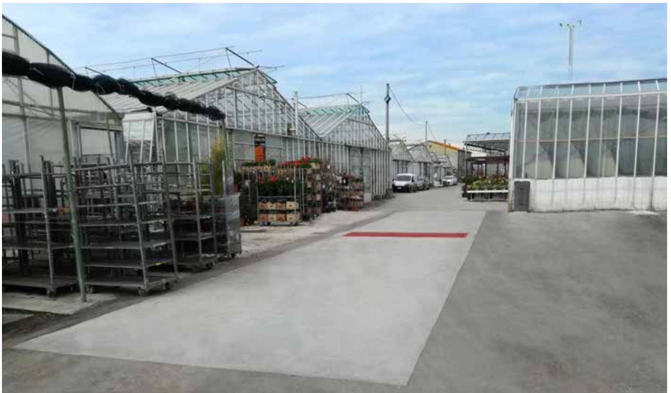
Example of cement spread foundation laying
