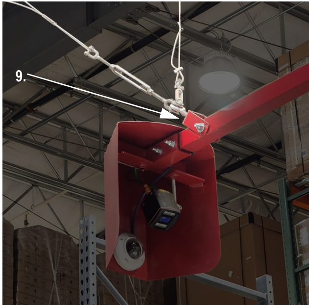
Figure 6. Turnbuckles to Hanger Assembly
