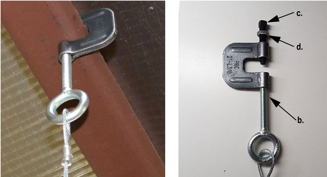
Figure 3. Beam Clamp to Roof Structure
