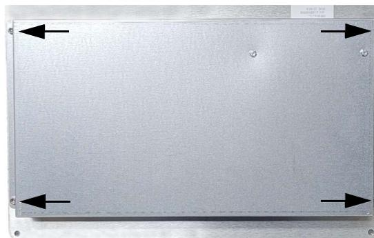
Figure 7. Ai-1 Indicator Cover Mounting Bolts
