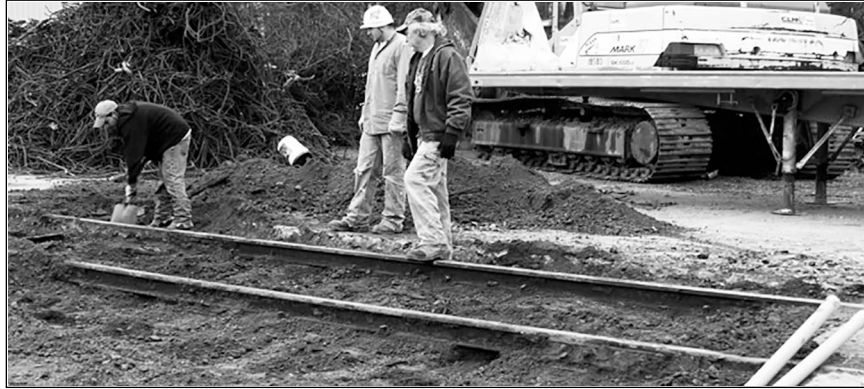
Figure 2-1. Existing Track Cleared of Ballast
