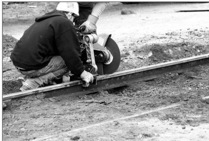
Figure 2-2. Cutting Existing Track
