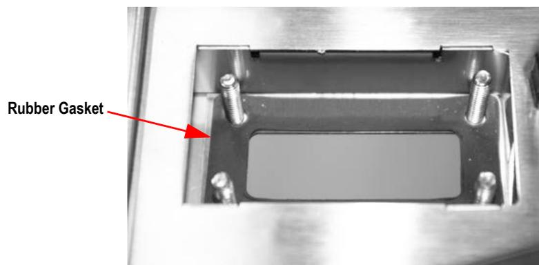
Figure 2-5. Rubber Gasket
