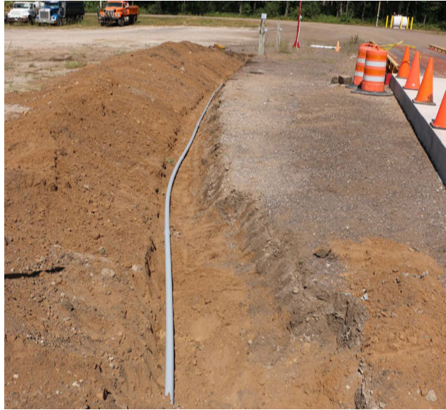
Figure 5-10. Trenched Cables
