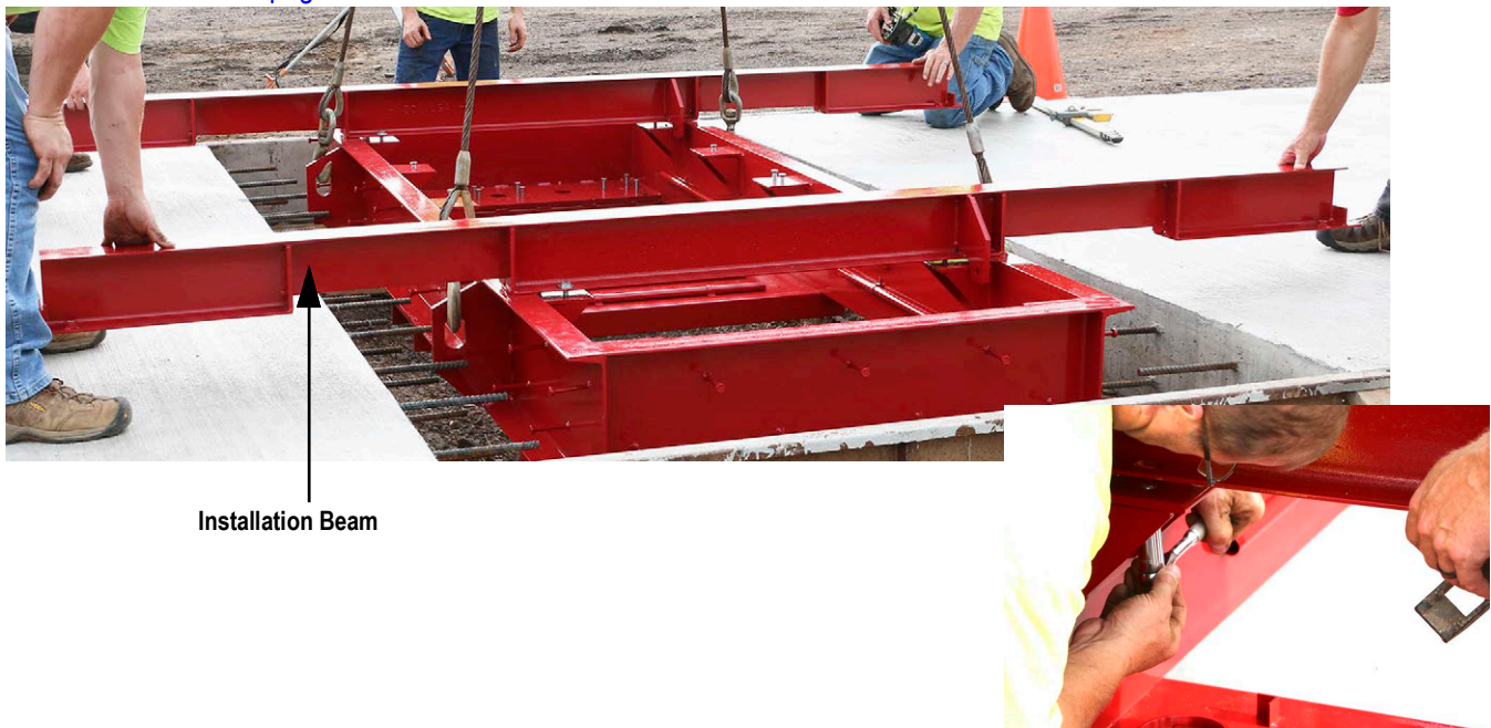
Figure 4-1. Fasten Installation Beams to Pit Frame
