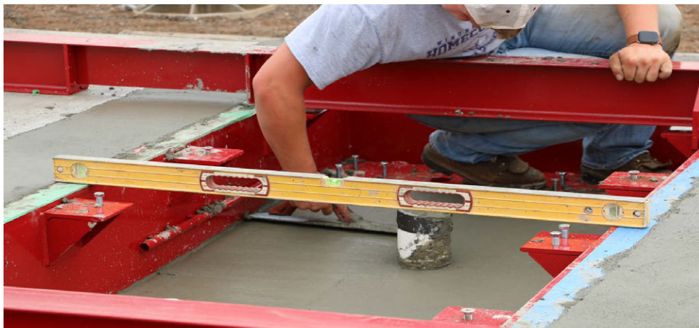
Figure 4-10. Taper Concrete
