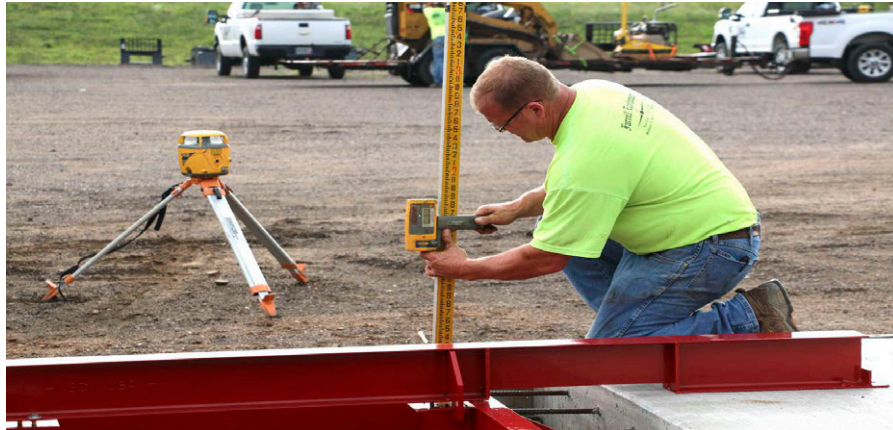
Figure 4-4. Ensure Pit Frame Is Level
