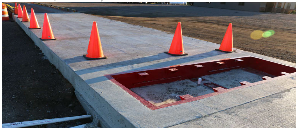
Figure 4-11. Pit Frame is Ready for Scale Deck
