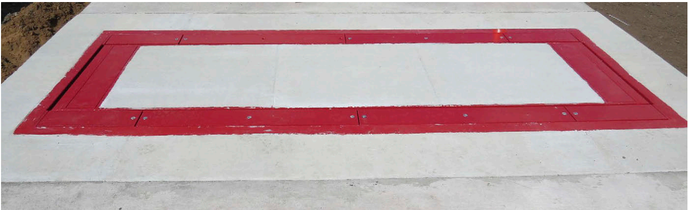
Figure 5-14. Weighbridge Installed in Pit Frame
