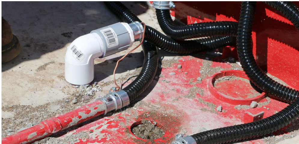
Figure 5-7. Connect Cabling to PVC Cabling Conduit
