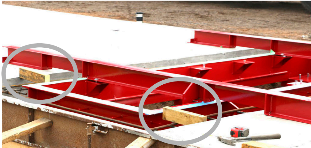
Figure 4-7. Ensure Pit Frame is Centered
