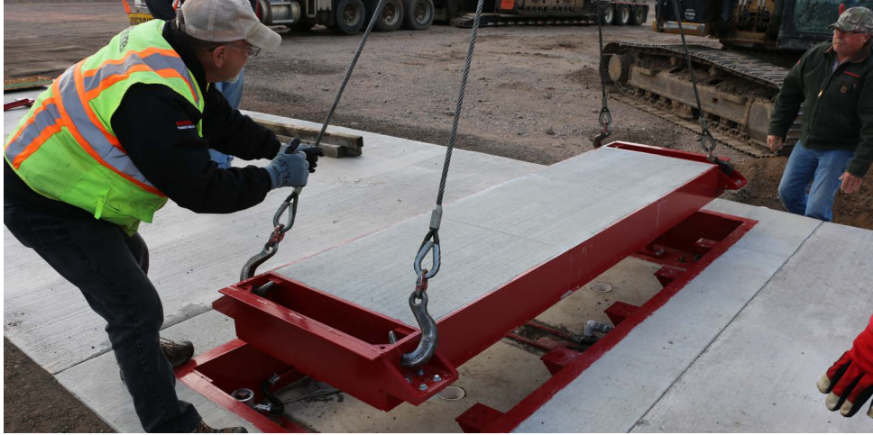
Figure 5-13. Lower Weighbridge Into Pit Frame
